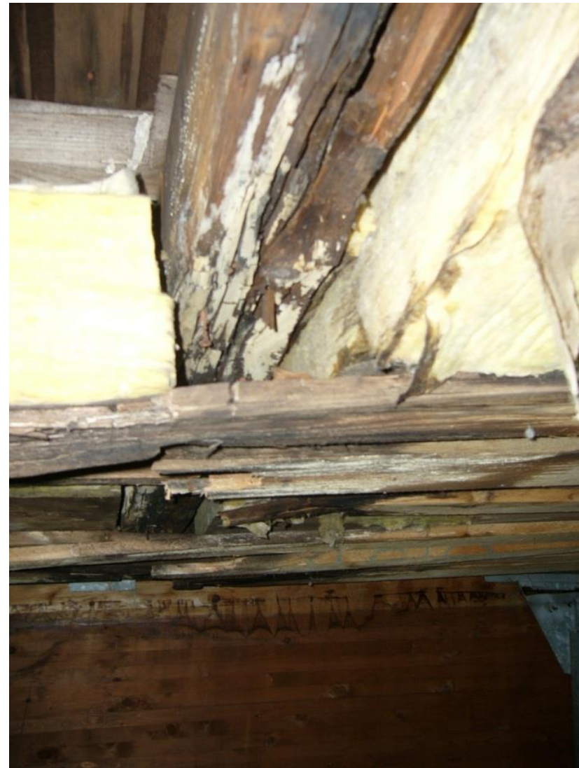
Rot inside the building structure
