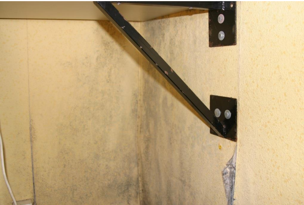
Mould (fungus) growth on the surface
